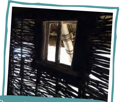
The wattle wall of the reconstructed roundhouse at Beeston. Note the window that was added to the design!
