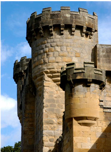
Close-up detail of the crenelated roof line around one of the castle's turrets.
