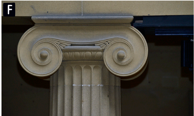
Scroll capitals at the top of pillars in the Pillar Hall hold up the floor above, as seen in classical Greek and Roman architecture.
