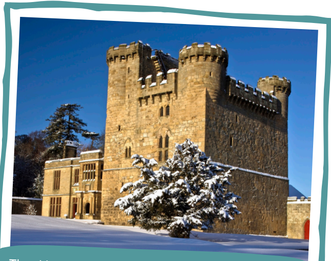
The oldest part of this building (on the right) was originally a free-standing pele tower. The manor house and west wing (to the left) were added later.
