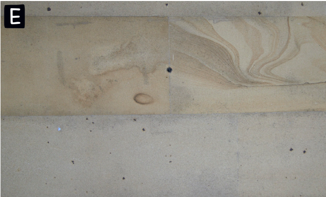
The bare stone blocks in the entrance hall are finely cut and fitted together without mortar – a building technique used in Greek temples.
