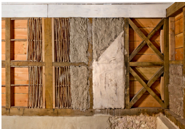
The wattle and daub wall, with wooden frame, on display in the Roman townhouse.
