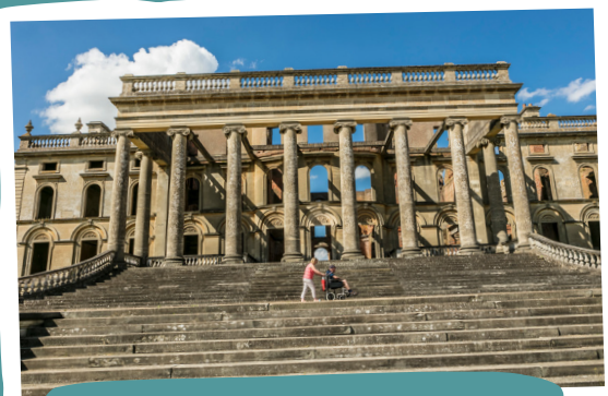
One of the porticos at Witley Court.
