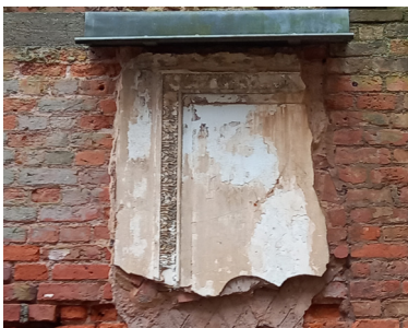
A section of plaster and putty decoration dating from the 1850s that survived the fire.
