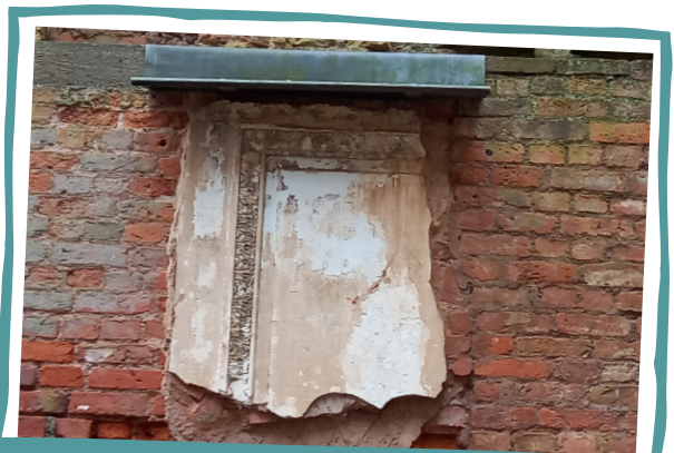
A section of plaster work decoration that survived the fire.
