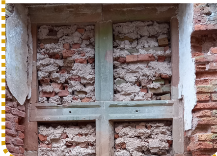
3 BLOCKED UP WINDOW
