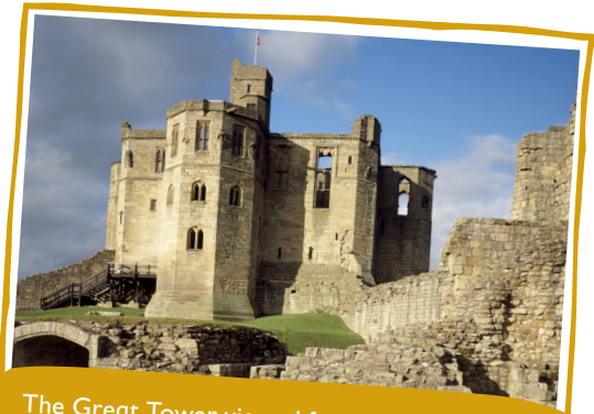
The Great Tower viewed from the gatehouse.
