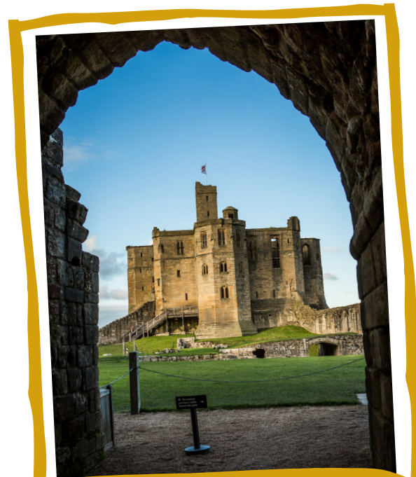
The Great Tower at Warkworth Castle, including the passage below the Collegiate Church, as seen from the inner bailey.
