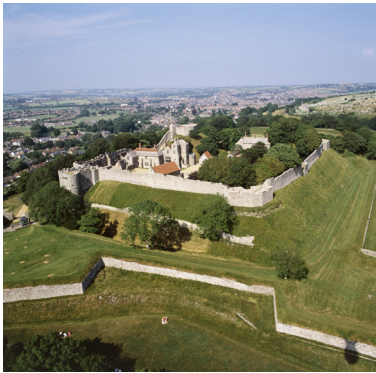
An aerial view of Carisbrooke Castle, showing how the castle is on high ground overlooking the town.
