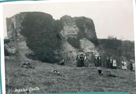
An early photograph of the inner gatehouse at Beeston showing visitors at the castle. The overgrown condition of the inner ward can be seen.
