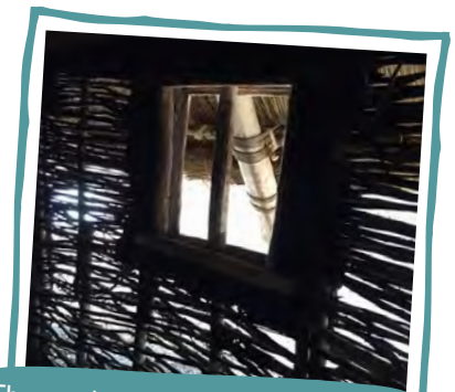
The wattle wall of the reconstructed roundhouse at Beeston. Note the window that was added to the design!
