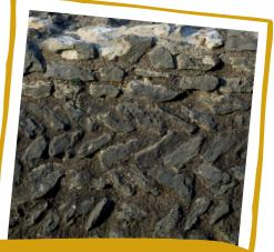
Most Norman castles were built quickly from earth and wood and rebuilt in stone later. Peveril Castle is unusual as it was built in stone first. The stones make a pattern called herringbone, as it looks like the bones of a fish.
