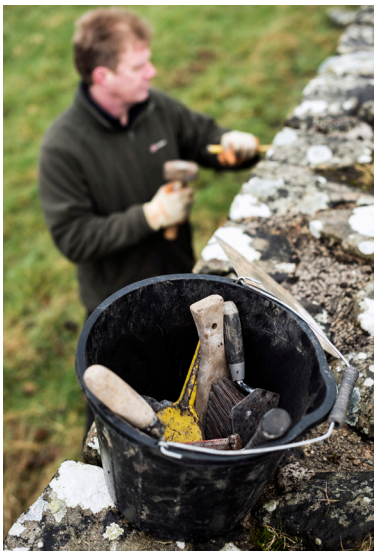
One of our experts maintaining the wall near Birdoswald Roman Fort.
