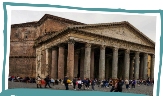
The Pantheon in Rome. Notice the first beam that rests on top of each of the columns. This is the architrave. The triangular part on top is known as the pediment.
