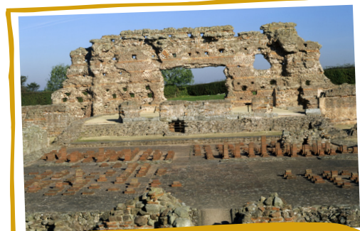
A view over the baths' heated rooms to the Old Work, the largest piece of free-standing Roman wall in the country, which used to separate the basilica from the bath suite.
