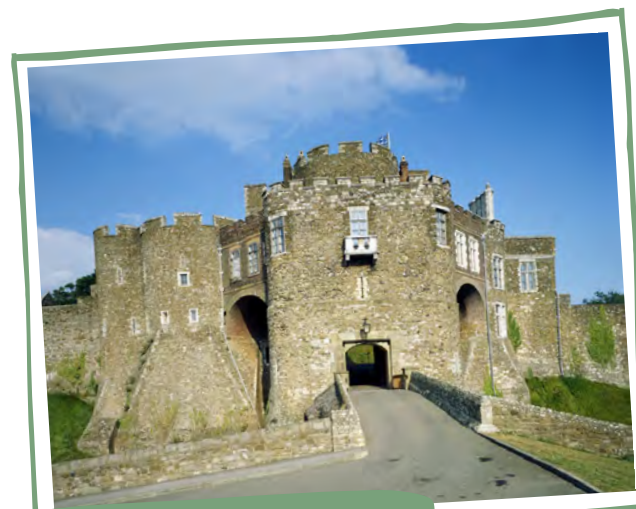
Constable's Gate von Dover Castle
