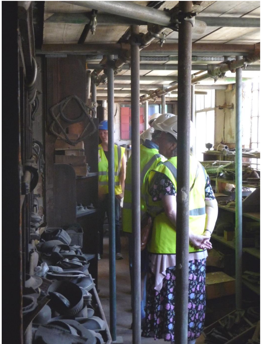
Fig. 8. Tours during building works. © English Heritage
