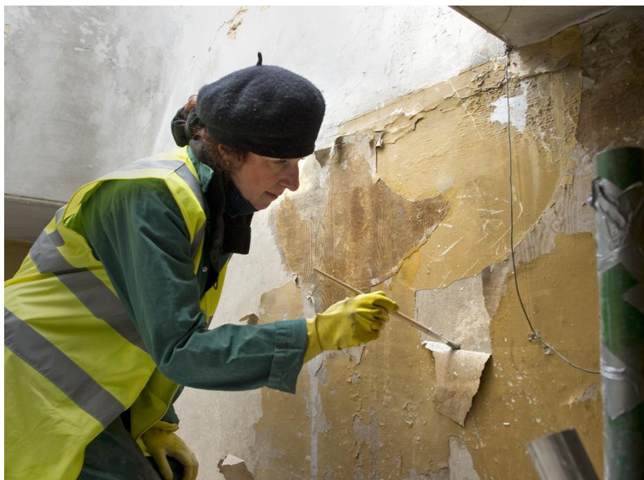
Fig. 6. Consolidation of interior surfaces. © English Heritage
