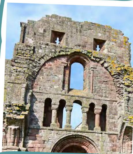
Arrow loops at the top of the West Front of Lindisfarne Priory church.
