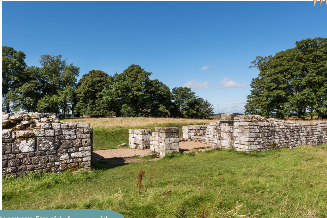
The east gate. Each of the four gates of the fort was designed the same way, with two arches and a supporting pillar in the middle.
