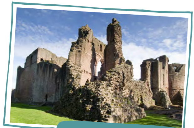
The north-west tower was severely damaged during the siege of 1646.
