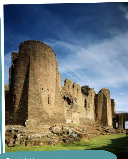
Goodrich's corner towers, battlements and arrow loops are typical features of medieval castles.
