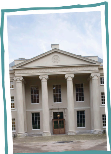
The Golden Ratio was used to calculate the ideal height of columns and the distance between them.
