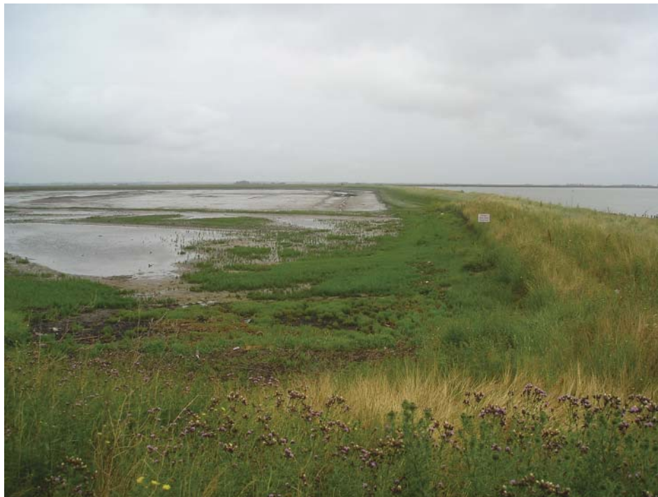
FIGURE 2 Wallasea Island, Essex: managed realignment. The formerly reclaimed area to the left of the sea wall (once maintained as grazing marsh and, later, arable) is now reverting to salt marsh and mudflat following sea wall breaching for realignment.
