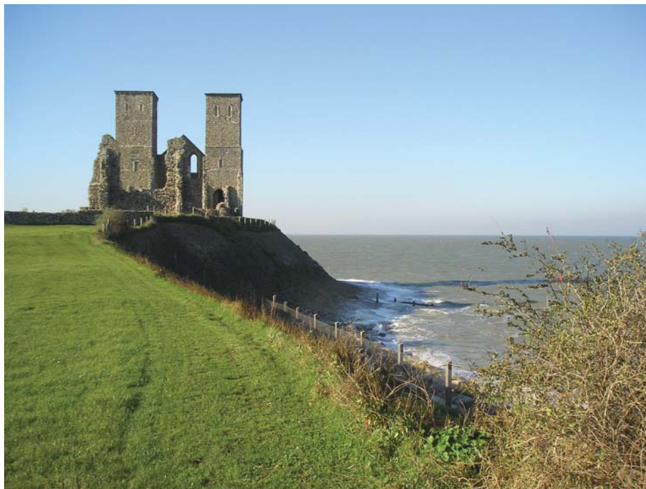
FIGURE 4 Reculver, Kent. The partly ruinous medieval church is on the site of a Roman fort of the Litus Saxonicum and an Anglo-Saxon monastery. The towers were only preserved because they act as a day-mark for mariners. The site is now heavily defended with rock-rubble armouring, without which it would erode rapidly, but will it be possible to sustain this through the twenty-first century?
