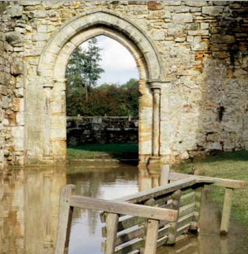
Severe storms and rainfall occurred across much of Kent and East Sussex in October 2000, causing wide spread damage at sites like Bayham Abbey, Bodiam Castle and over 800 properties in the centre of historic Lewes.
