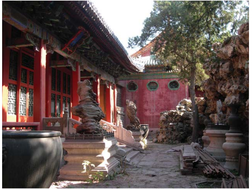
Beijing: the exquisite Juanqinzhai (Studio of Exhaustion from Diligent Service) was the first building in the Emperor Qianlong's magnificent retirement garden to be restored in a joint partnership between the Palace Museum and World Monuments Fund.
