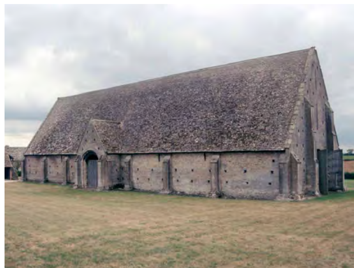
Fig 1. Barn, Great Coxwell, Oxfordshire. The safe storage of grain crops, especially fresh off the fields, was always essential to the great estates. This massive limestone barn was built by the Cistercian monks of Beaulieu Abbey about 1246. Inside, aisle posts alternate with a form of base crucks. Listed Grade I.
