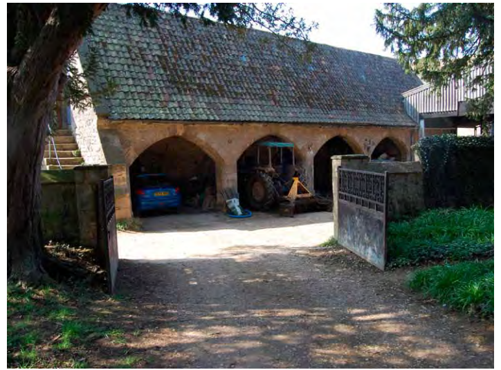
Fig 5. Cartshed with granary over, Frocester Court, Gloucestershire. In the Middle Ages Frocester was a great monastic estate, and a thirteen-bay barn survives from that time. About 1850, when ranges of new buildings were constructed by an improving farmer, their styling was deliberately medieval, and the quality high. Listed Grade II.
