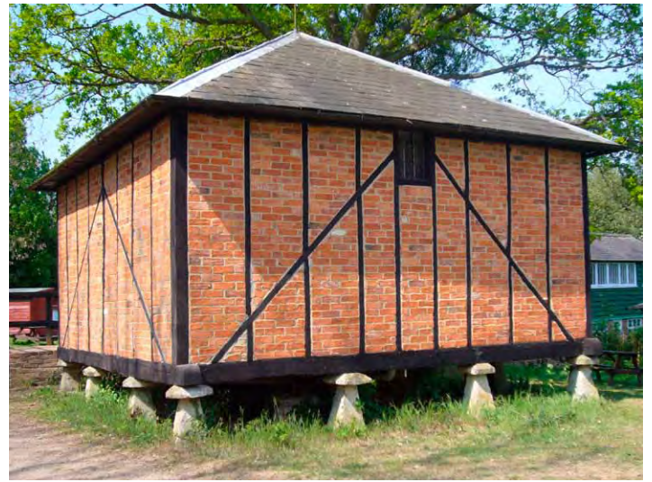
Fig 3. Granary, Pike's Farm, Haversham, Buckinghamshire (now at Chiltern Open-Air Museum, Chalfont St Giles, Buckinghamshire). Granaries, used to store heavy sacks of grain, are necessarily robust buildings; that, coupled with their elevation off the ground which reduces rot, means they tend to survive relatively well. Even late examples, such as this of about 1840, tend to be firmly in local vernacular traditions.
