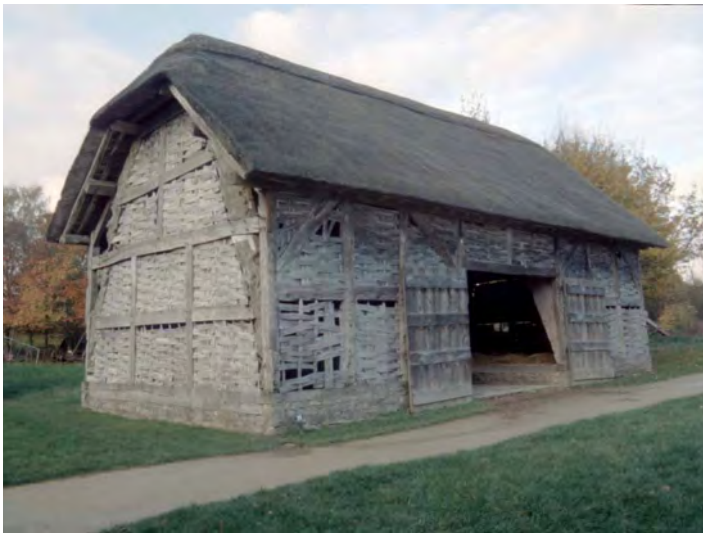
Fig 2. Cruck-framed barn, Cholstrey Court Farm, Leominster; Herefordshire (now at the Avoncroft Museum, Bromsgrove, Worcestershire). While sharing features like large cart doors and threshing floors, pre-nineteenth-century barns have a strongly vernacular character. This sixteenth-century example reflects the predominance of timber-framed building – here the frame is of black poplar – in the Welsh Marcher counties. Removal to a museum does not preclude listing. Listed Grade II.
