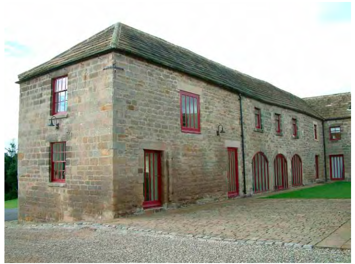
Fig 16. Stocksfield Farm, Hexham, Tyndale. A nineteenth-century planned farmstead successfully converted to multiple business uses. Listed Grade II.
