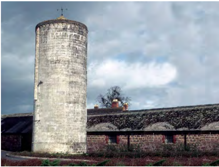
Fig 12. Concrete silo, Holme Lacy, Herefordshire. In England, the move from hay to silage – cut grass stored in an air-tight container – began in the 1880s, although it was only during the Second World War that the movement really took off. This American-style concrete silo of 1912 was therefore in advance of the general trend.
