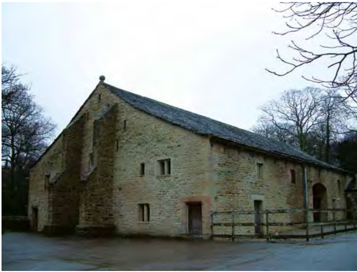
Fig 4. Combination Barns, incorporating areas for crop processing alongside housing for cattle, are strongly characteristic of Lancashire (as here) and the north-west.
