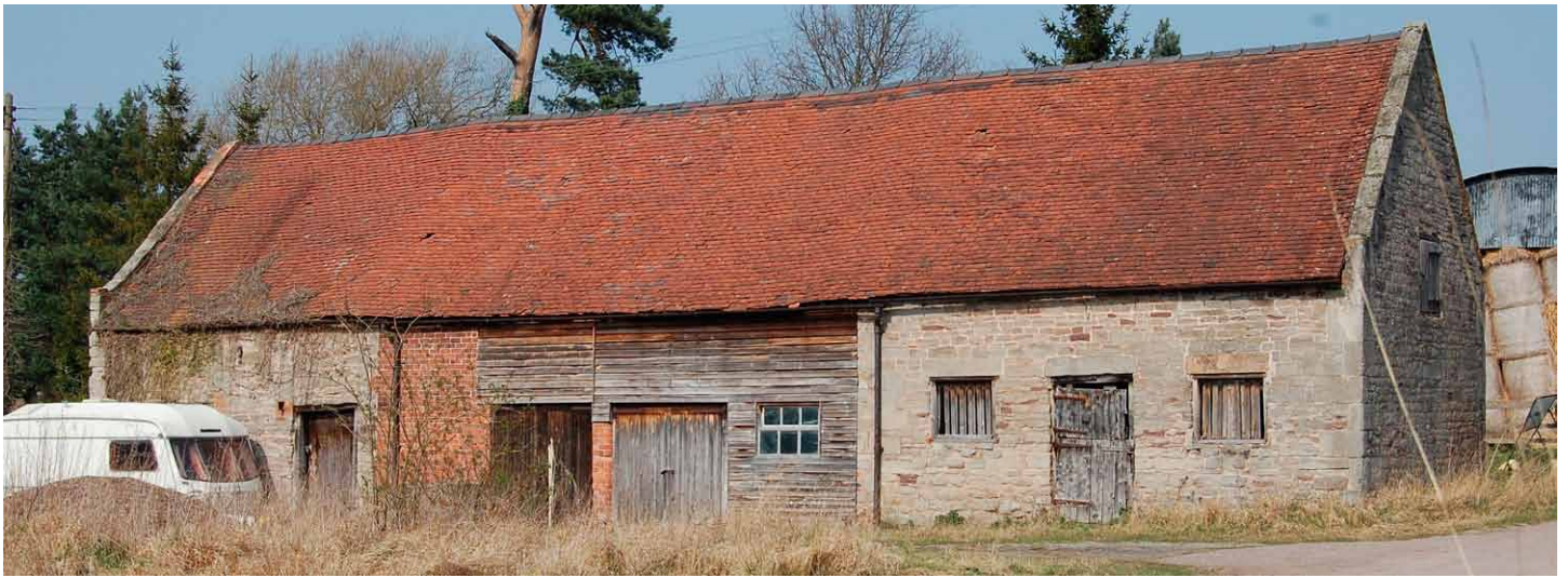
Fig 14. Multi-functional agricultural building, Morville, Shropshire. This unlisted structure illustrates how historic agricultural buildings see adaptation and change over the centuries. Even so, they tend to remain legible. Here it is immediately obvious the right-hand end,
