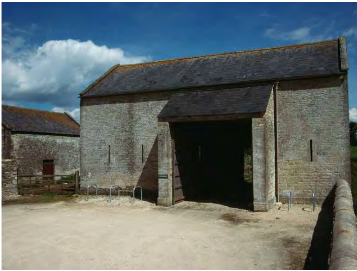
Fig 15. Ewepen Farmbuildings, Sherborne, Gloucestershire. In the Cotswolds, where stone was plentiful, the vernacular tradition lingered much later than in those parts of the country where brick was gratefully adopted. This barn, and the adjoining shelter, are of about 1860. Although of relatively late date the farmstead makes a very strong contribution to its locality. Listed Grade II.
