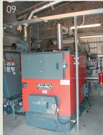
At Aske Hall, near Richmond in North Yorkshire, wood-chip boilers are being progressively installed as more efficient and environmentally friendly replacements for traditional heating systems. 08: Aske Hall stableyard, 09: wood-chip boiler; 10: traditional building used as a hopper for the wood chip. © Historic House Association
