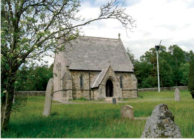
03 Dalehead Church (Bradford Diocese). The chapel and Heritage Centre are powered by wind turbine. The graveyard is a Biological Heritage Site with more than 130 species of upland meadow plants. © Mr John Parry
