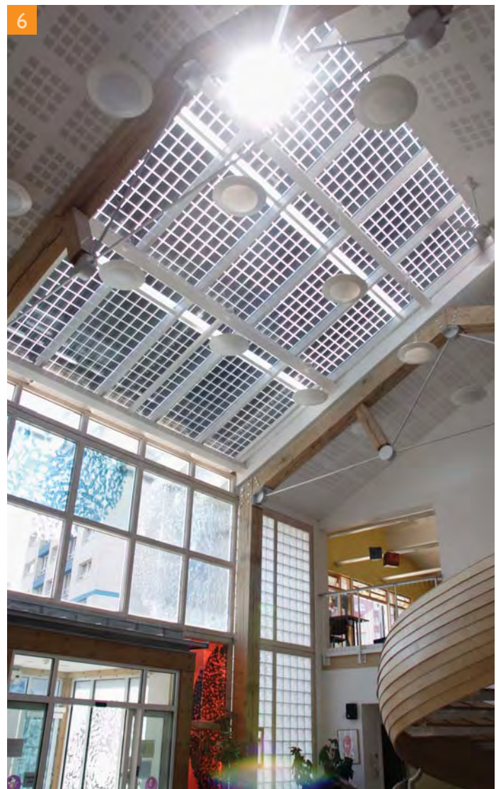
PVs integrated into glass (Photograph courtesy of Solar Century)
