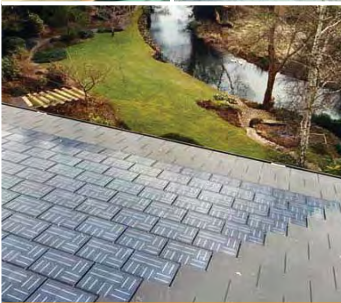
Top left: Close up of PV slate installation. Top right: Individual PV slate. Bottom: Roof covered with PV slates. (Top left and bottom: Photographs courtesy of Sunslates Limited. Top right: Photograph courtesy of Solar Century.)
