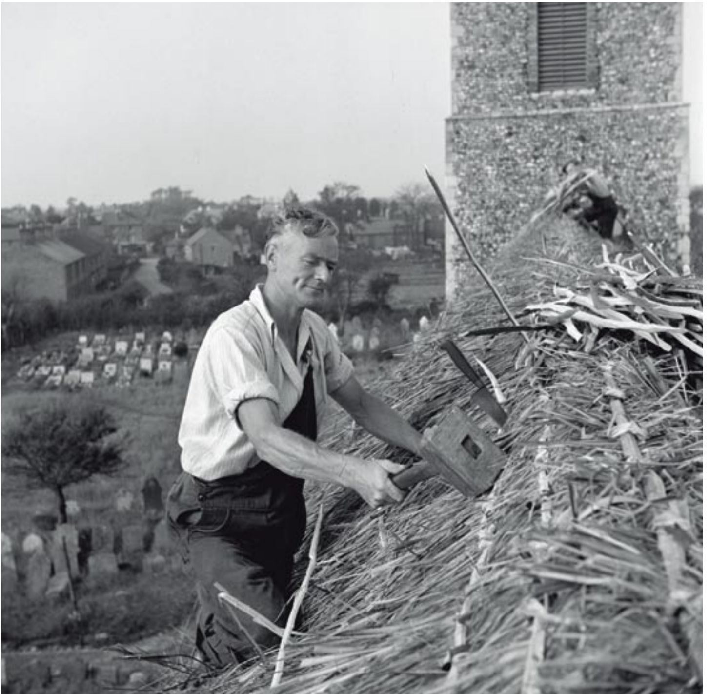
St Margaret and All Saints Church, Pakefield, Suffolk (Grade II*). A reed thatcher carrying out repair work on the church roof, photographed by Hallam Ashley in 1949.
