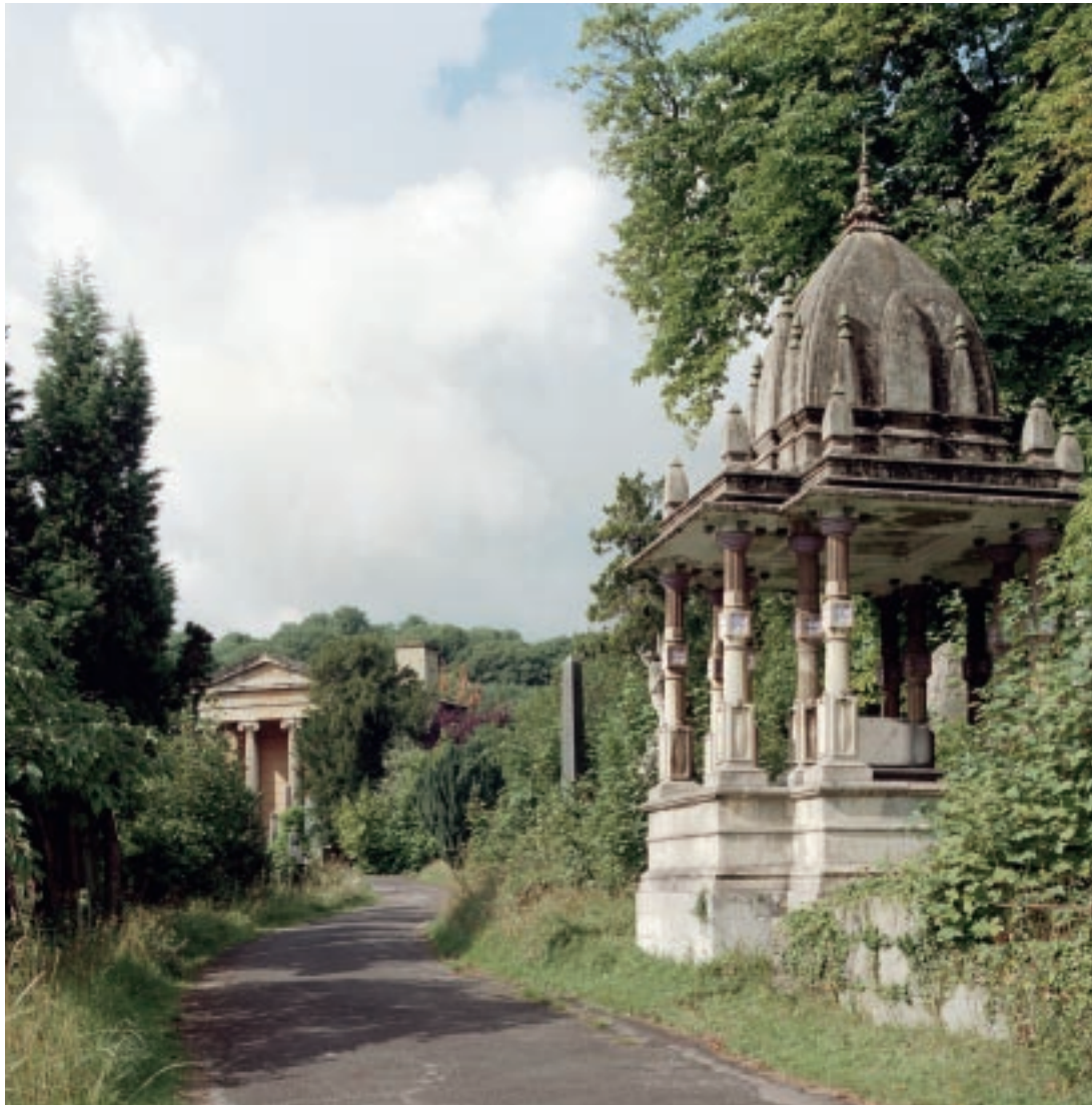
The Grade II* listed monument to Raja Rammohun Roy – a Hindu reformer and thinker who died in Bristol 1833 – designed by William Prinsep. Beyond is the Dissenters' Chapel, with a Greek Ionic portico designed by Charles Underwood about 1840. Arnos Vale Cemetery, Bristol (Grade II*), was laid out by Bristol nurserymen James Garraway and Martin Mayes
