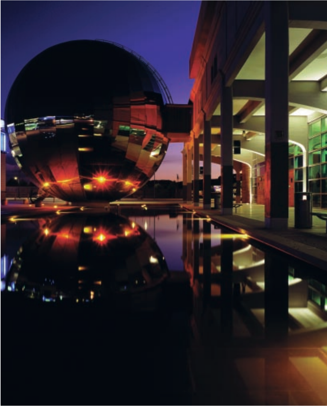
The Planetarium by night, with glass bridge to main building. The final concrete half arches meet pillars with original metal cladding showing the level of a former station platform
