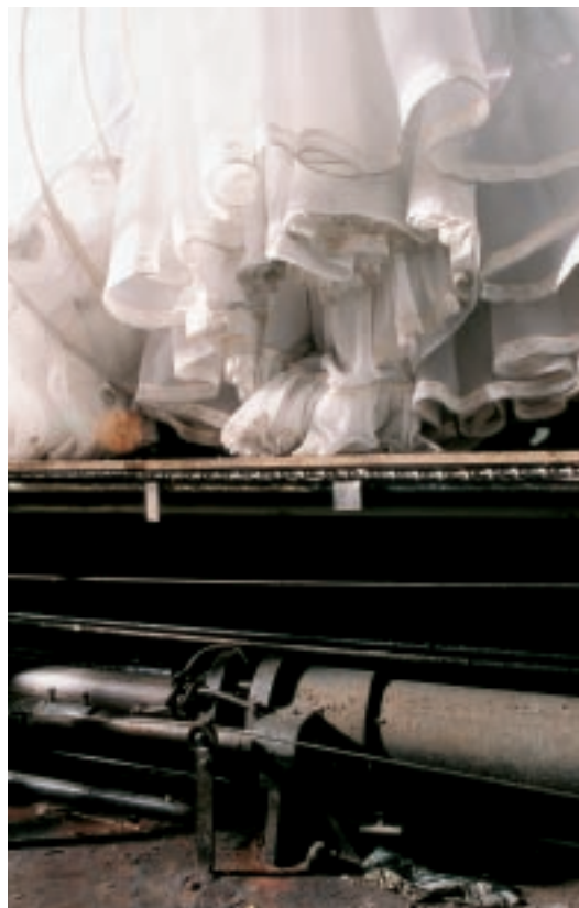
Sub-stage at the London Palladium Theatre, a view of the hydraulic ram used to raise the safety curtain; above, the frills and furbelows of theatrical costume from the production of The King and I
