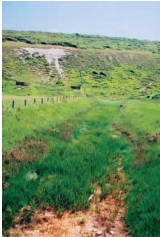
Section of unfilled anti-tank ditch, with pillboxes behind, at Cuckmere Haven, East Sussex
