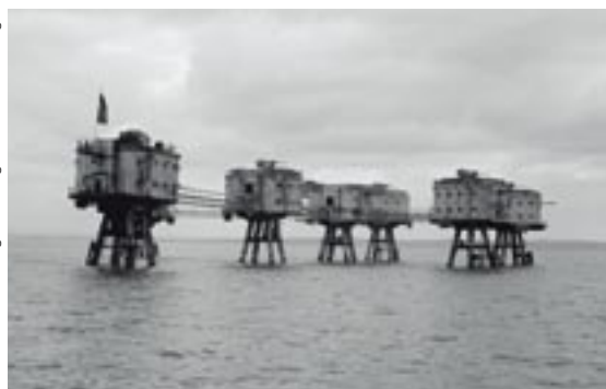
Maunsell Forts, Shivering Sands, somewhere between Southend-on-Sea and Margate. Designed by GA Maunsell, these army forts were erected for defence during 1941–2.
