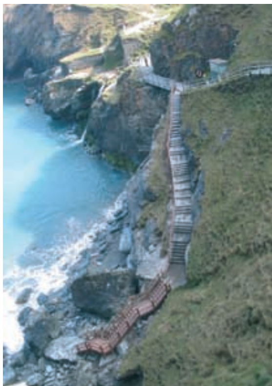
Tintagel Castle, Cornwall: view of the new beach steps installed in 2003 to improve visitor access. The work was carried out as part of a wider Tintagel Regeneration Project part-funded by the European Regional Development Fund (Objective 1) and in partnership with Cornwall County Council.
