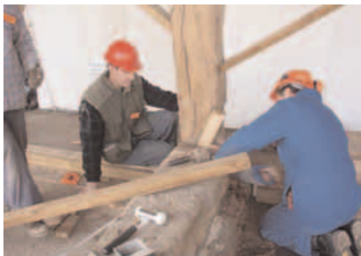
Trainees on the 2004 'Heritage Crafts' training programme replacing the sole plate of a 14th-century Grade II listed timber-framed barn in Terling, Essex.
