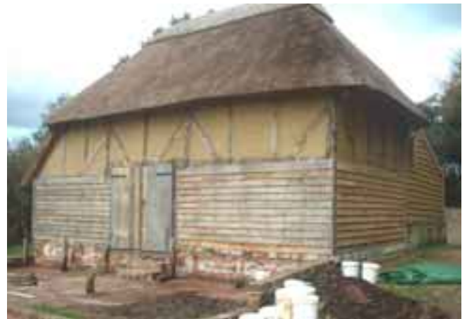
Known from parish records to have been blown down in 1667–78 and rebuilt in 1702, this building was found to be a typical Sussex timber-framed barn underneath the external accretions. Using only the building's archaeological evidence, the HLS grant-aided works reinstated the thatched roof and wattle-and-daub infill. The restoration won a Sussex Heritage Award and the barn is now used to shelter participants attending wild-flower seed-harvesting demonstrations on the estate.
