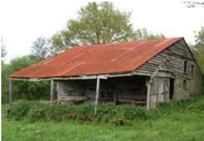
Known from parish records to have been blown down in 1667–78 and rebuilt in 1702, this building was found to be a typical Sussex timber-framed barn underneath the external accretions. Using only the building's archaeological evidence, the HLS grant-aided works reinstated the thatched roof and wattle-and-daub infill. The restoration won a Sussex Heritage Award and the barn is now used to shelter participants attending wild-flower seed-harvesting demonstrations on the estate.
