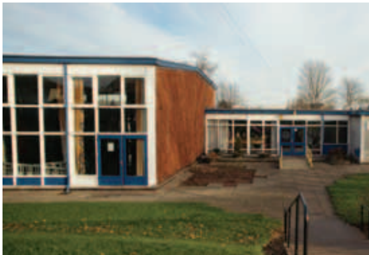
Intake School, Mansfield, 1956, Nottinghamshire County Council Architect's Department. Called the 'Rock 'n' Roll' school for its ability to ride mining subsidence, this was the first school to be built using the CLASP system and is the only post-war school in the county to be listed.
