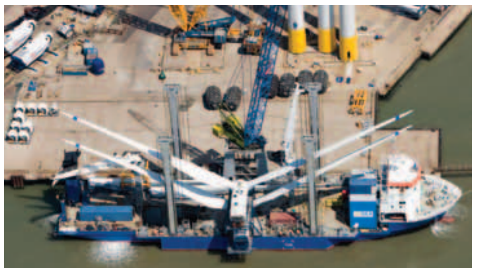
Off-shore wind-farm construction at Lowestoft, Suffolk. © English Heritage
