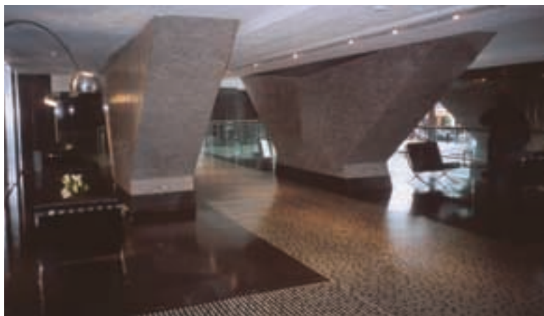
Centre Point, The mezzanine entrance lobby with mosaic-clad pilotis and distinctive paving.
