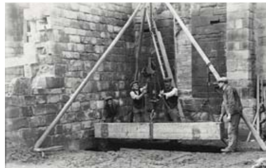
Fig. 47 (right, below): Photograph of 26 March 1930 showing underpinning operations in the east range
