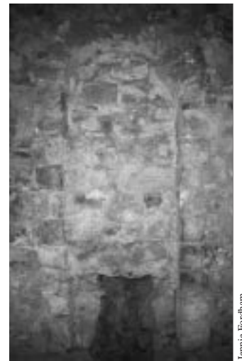
The blocked doorway
