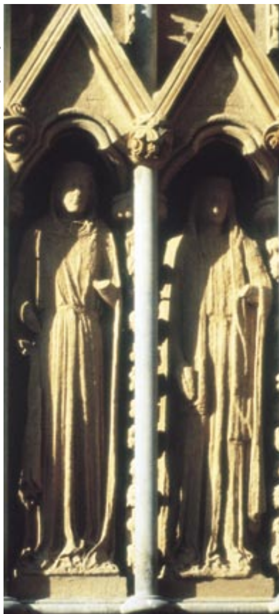
Wells Cathedral, Somerset, where extensive consolidation with calcium hydroxide has been carried out.
