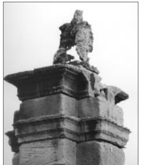
Pupils can record the badly eroded griffin that remains on the top of the gatepost at the entrance to the courts. Pupils can design a new griffin, researching what the griffin might have looked like and making models in clay, modroc or other suitable modelling materials.
