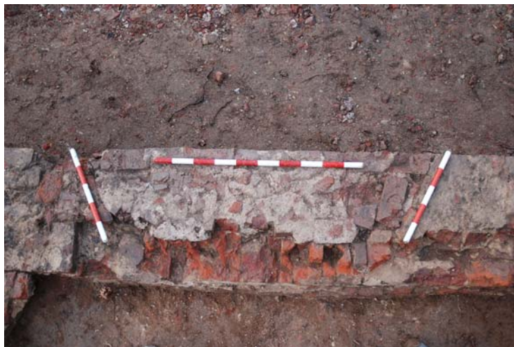
Photograph showing the blocked basement window opening at the front of the southern range of the Jacobean House (1m and 2 x 0.5m scales)
