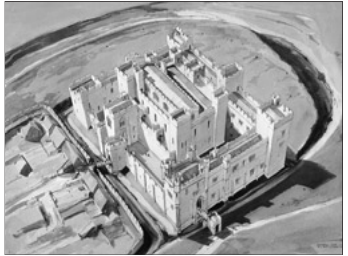
The keep is one of the largest in England measuring 32 metres by 23.8m with walls 3.6m thick, 20m high and built of ashlar with a rubble core. These artist's impressions show how the keep sustained its business and domestic role while the accommodation around the curtain walls was substantially improved.
