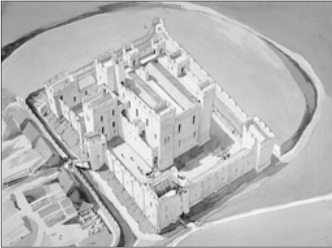
The keep is one of the largest in England measuring 32 metres by 23.8m with walls 3.6m thick, 20m high and built of ashlar with a rubble core. These artist's impressions show how the keep sustained its business and domestic role while the accommodation around the curtain walls was substantially improved.
