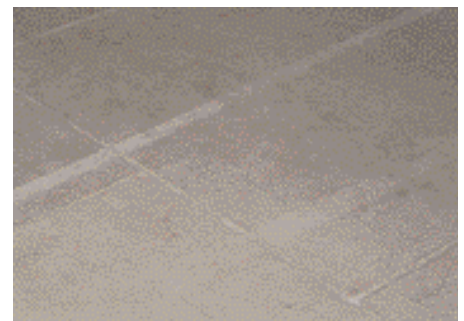
Marks left from the removal of tape attaching druggetting to the floor. [©Nicky Ingram]
