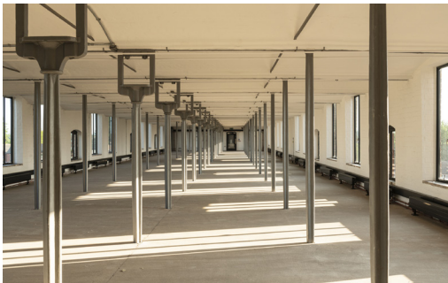
The columns that form part of the iron frame are visible in this photo of the third floor of Shrewsbury Flaxmill Maltings.
