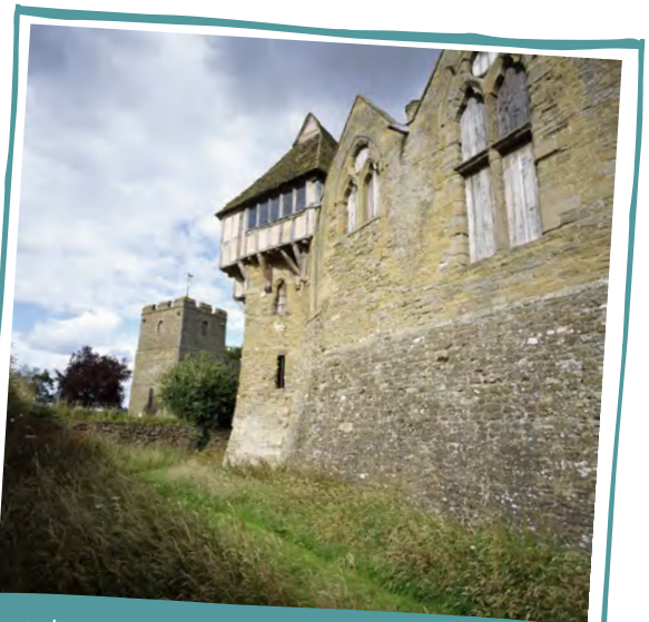
It's not clear whether the moat at Stokesay was originally filled with water, or kept dry. Either way, it would have been an effective barrier against animals and low-level crime.
