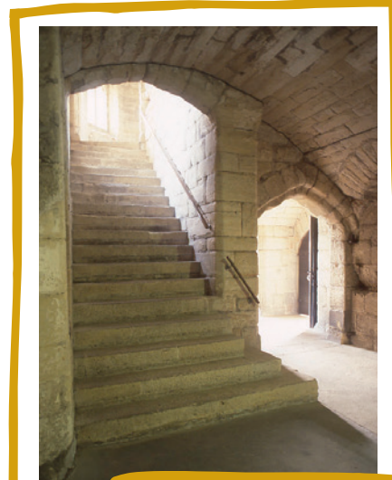
The staircase leading from the entrance hall to the lobby.
