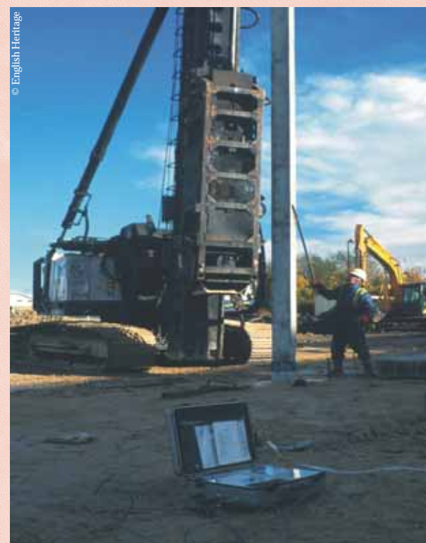
I contribute to a government funded project examining the effect of loading on archaeology, as well as looking at the effects of piling.
