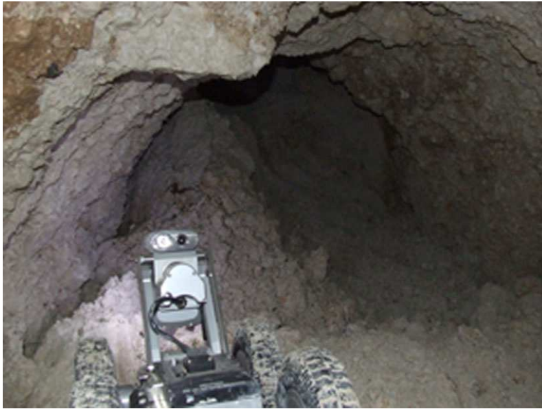
The Rover filming the tunnel
