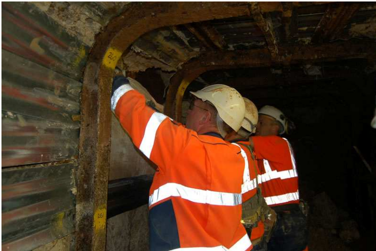
Engineers checking the tunnel sides
