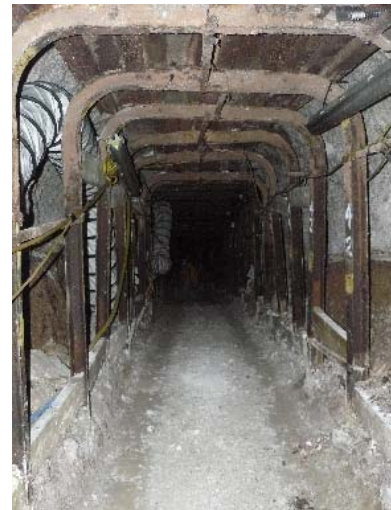
Figure 1: Tunnel conditions 7 th Jan 08
