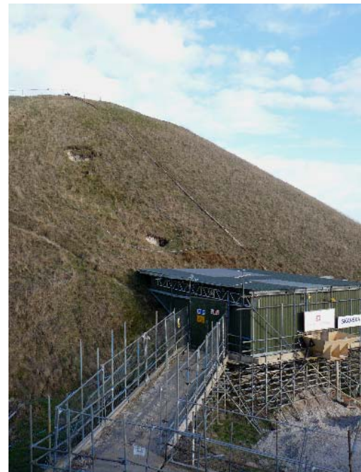
Figure 2: hill side collapse features
