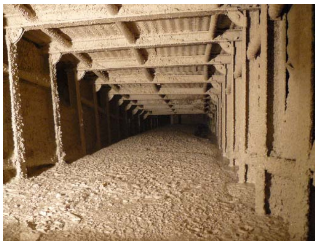
Figure 1: Paste backfilling of the 'Kirkbride' tunnel
