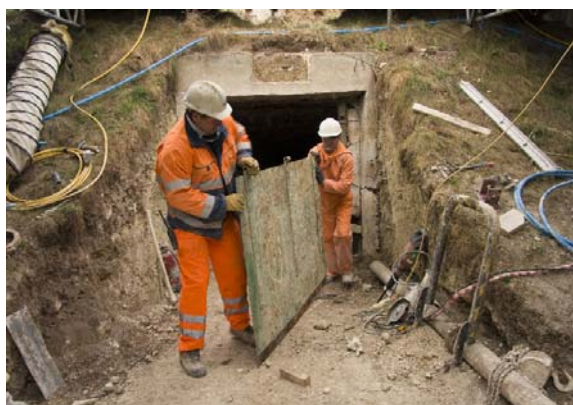
Figure 2: removal of the 1968 door
