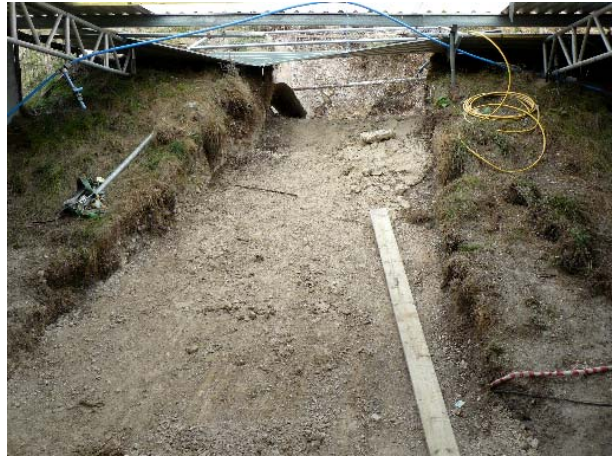
Figure 4: bank of chalk emplaced at the old tunnel entrance
