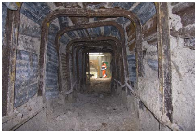
Figure 1: the final section of tunnel prior to filling
