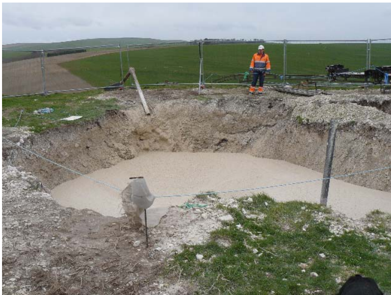
Figure 5: hilltop void infilling progress
