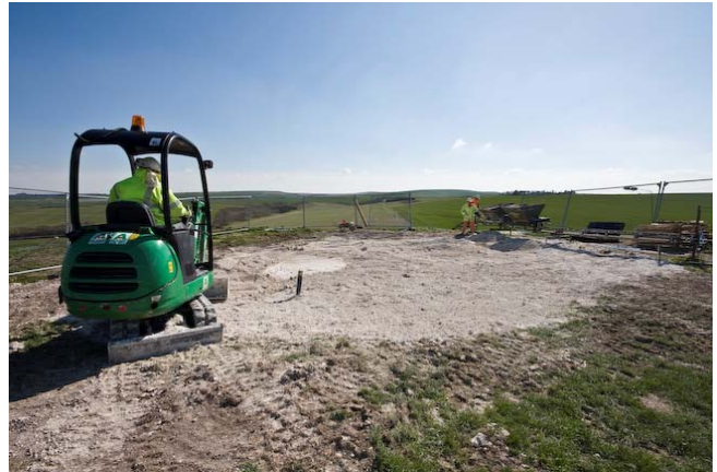
Figure 1: completing the hilltop works
